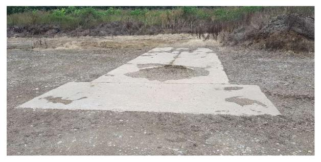
Concrete slab assumed capping decommissioned well
